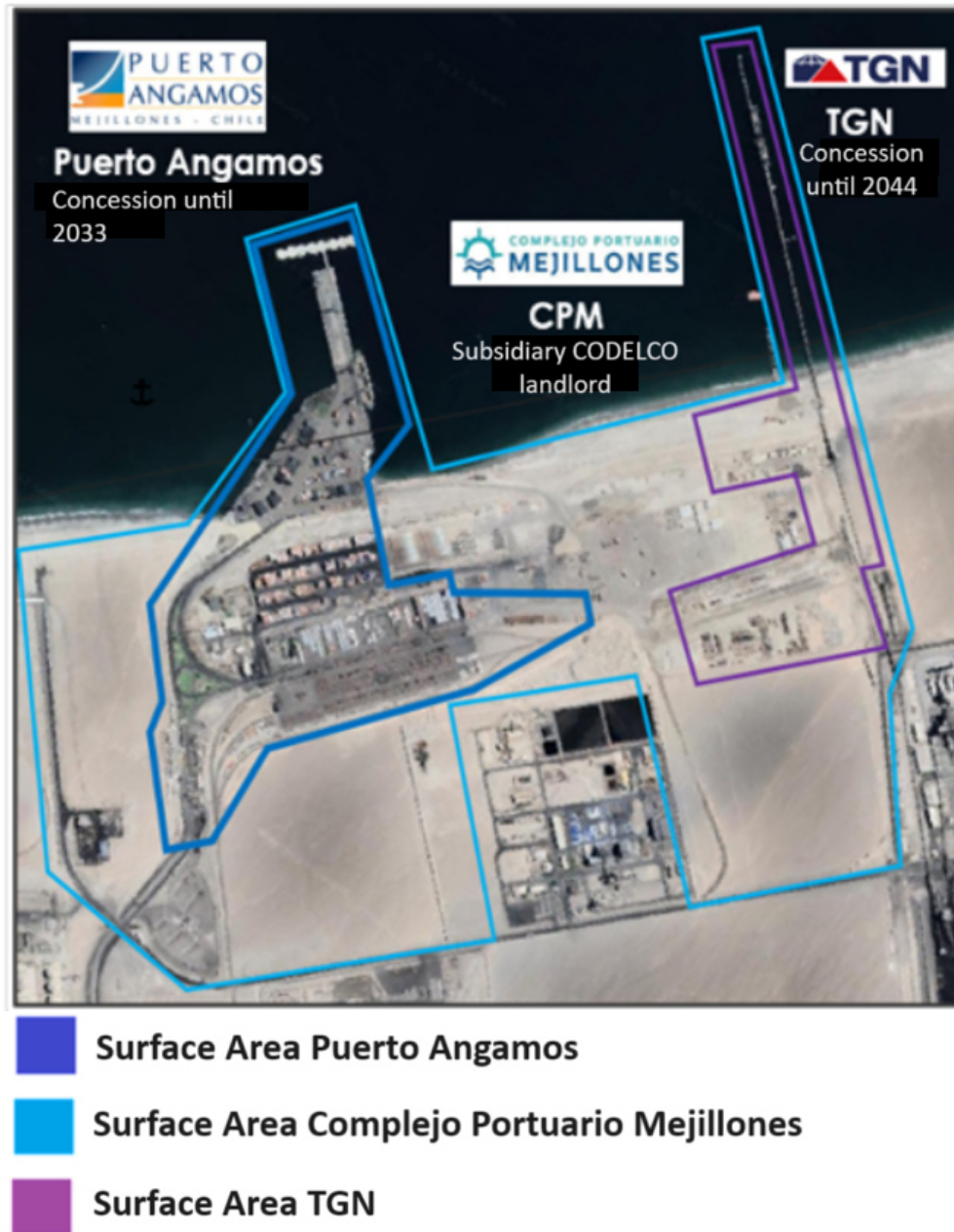
Figure 13. Terminals of the Port Complex of Mejillones.
