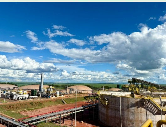
Figure 1 - The image shows Cocal's production site in Paraguaçu Paulista- SP, featuring biogas facilities and CO 2 capture technology. Photo: GIZ
